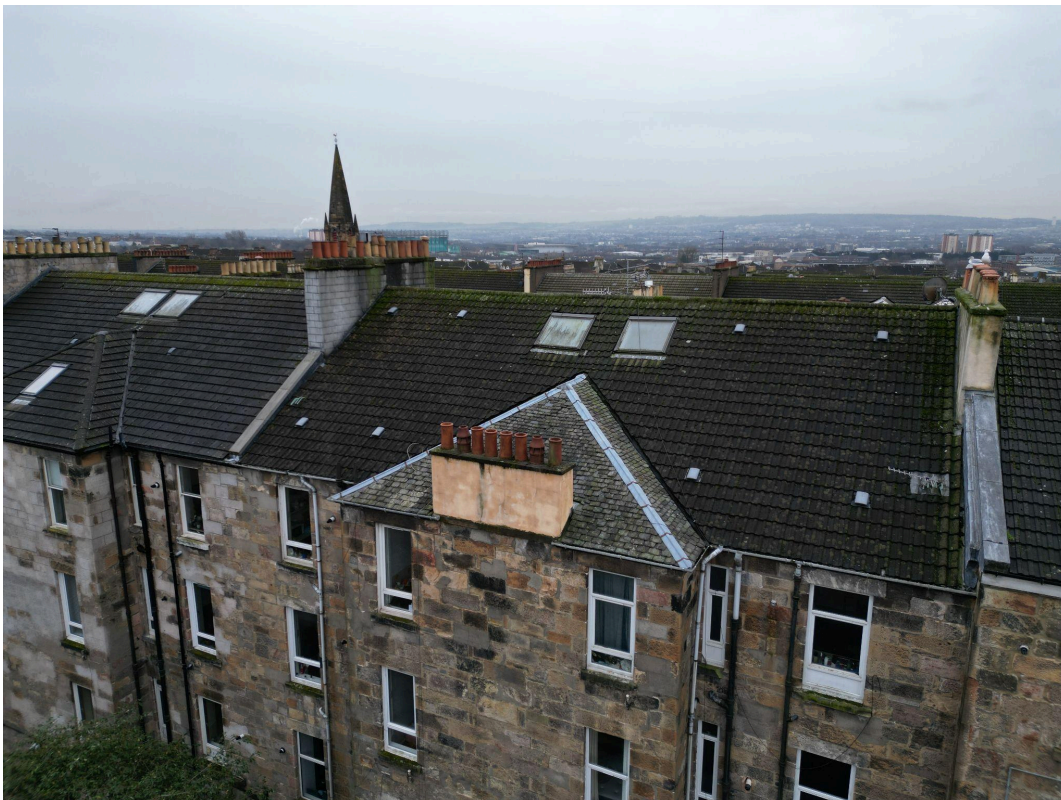
Figure 4.1: Drone photograph of rear elevation and roof.
