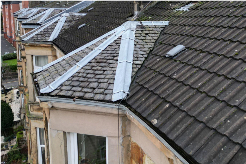
Figure 4.2: Front bay window and guttering.
