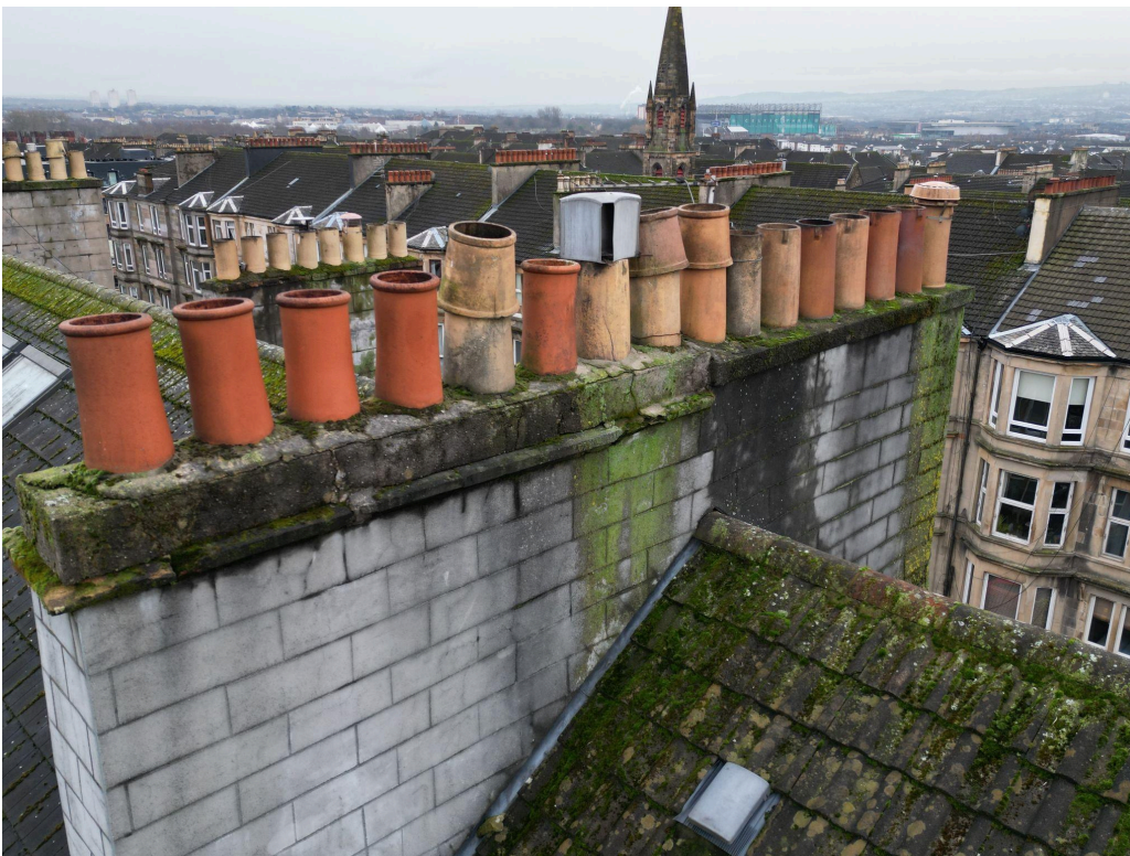
Figure 4.3: Chimney pots on the east wallhead.
